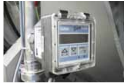
Exact water supplies with inductive-type flowmeters
